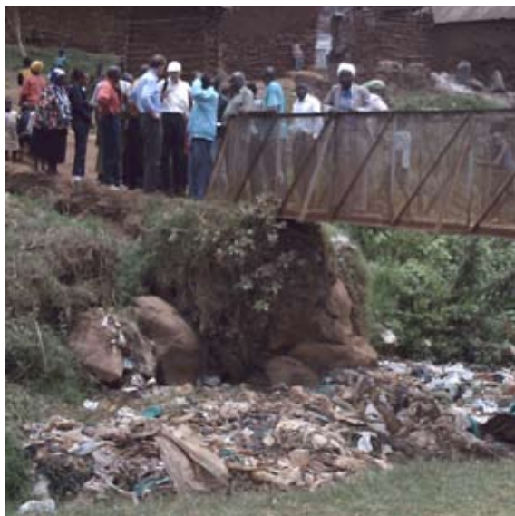
Poor sanitation facilities - a garbage pile
